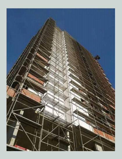
Exterior walls: Made of hollow brick in a single wall with thermal insulation using 8 cm polystyrene chemically bonded with a special glue and mechanically with dowels, and in addition to mesh.
